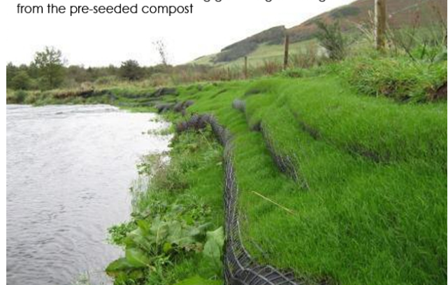
6 weeks after installation showing good vegetation growth from the pre-seeded compost
